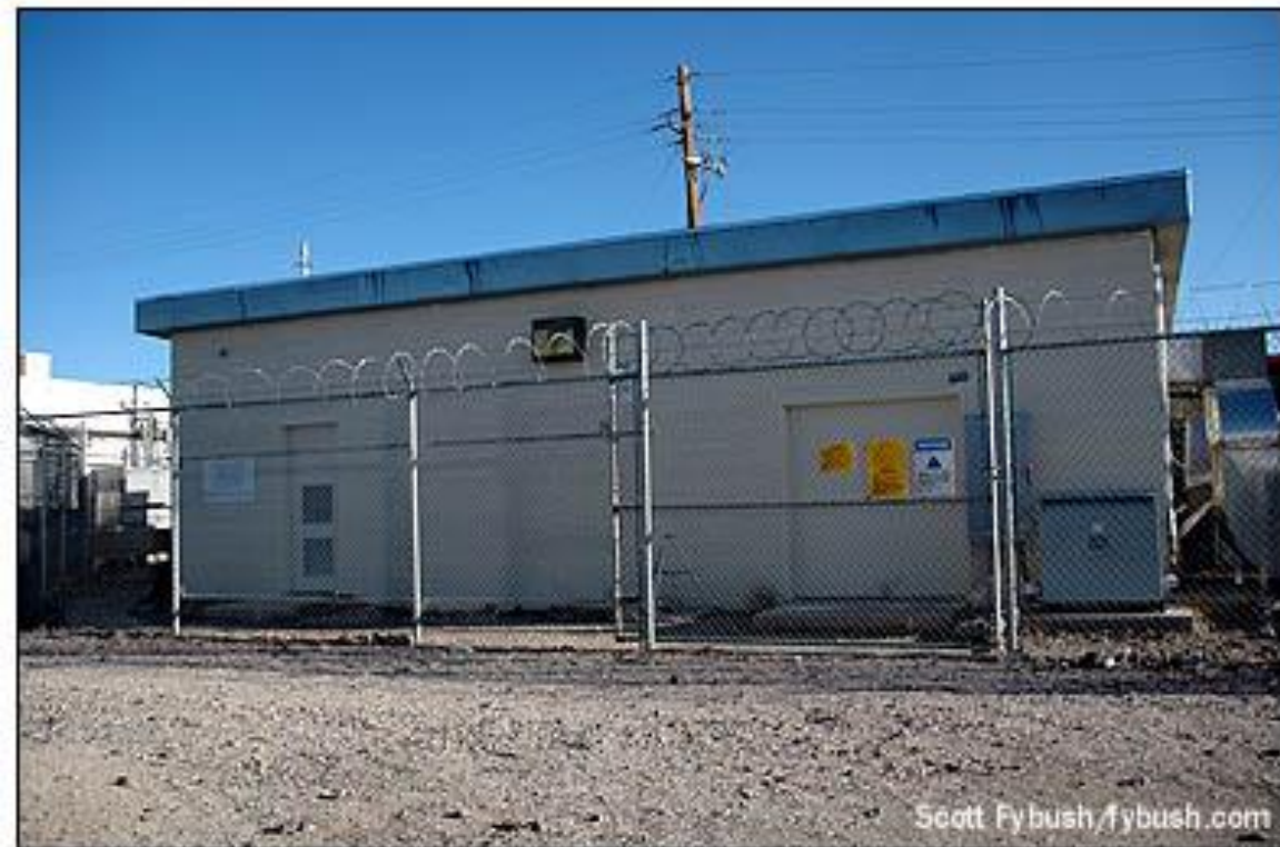
KTNV's transmitter building
