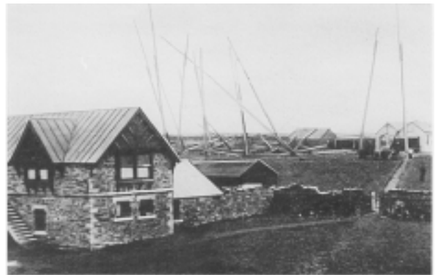
31 The effect of bad weather on the first Poldhu aerial
